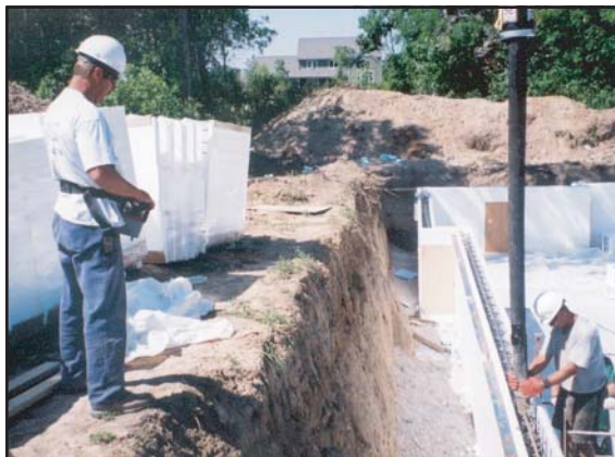
The Ruff-Neck™ Reducing Hose maintains a smooth, controlled flow
